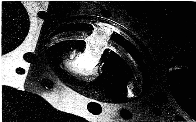
Repaired area after finish grind of repair material.
